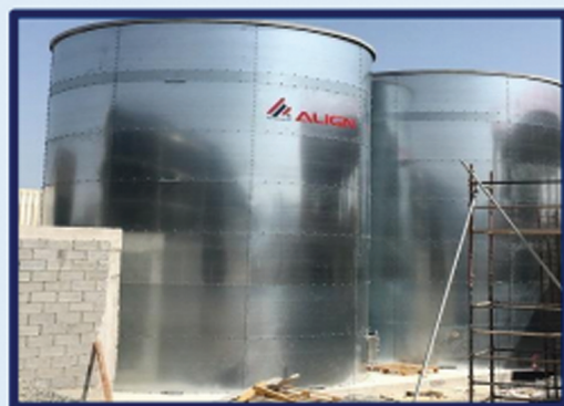
WAREHOUSE, OFFICE FOR M/S RAKHA AL KHALEEJ, JAFZA, DUBAI
